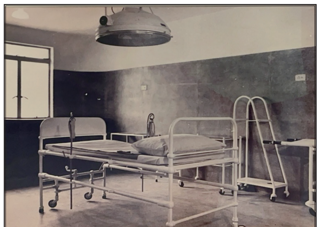
Figure 6. The setting of a labour ward.
