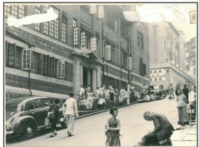
Figure 3. The main entrance of the old Tsan Yuk Hospital.
